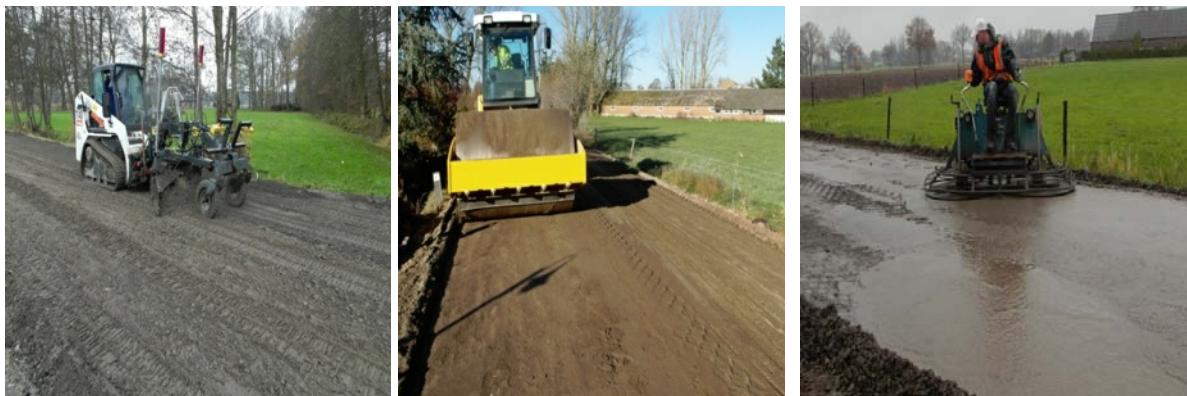
Figure 7.13 Levelling, compaction and polishing surface
