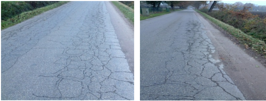
Figure 7.5 Observed distress in the existing asphalt pavement
