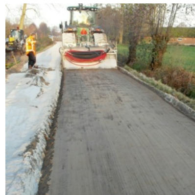
Figure 7.11 Applying cement and dry mixing
