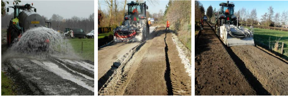
Figure 7.12 Adding water and wet mixing
