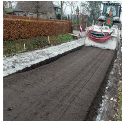
(c) Mixing Rc and in-situ sand
