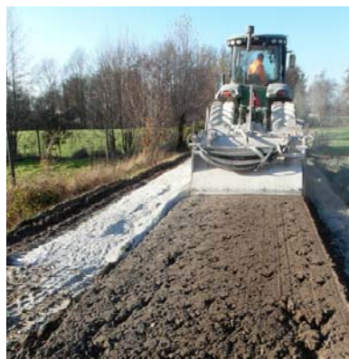
Figure 7.11 Applying cement and dry mixing
