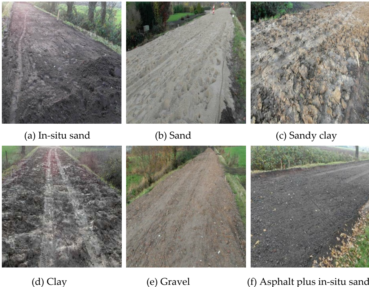
Figure 7.9 Preparation of the layers of soil materials
