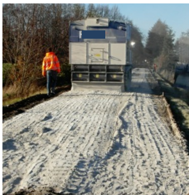
Figure 7.11 Applying cement and dry mixing
