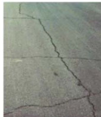
(b) Wide reflection crack
