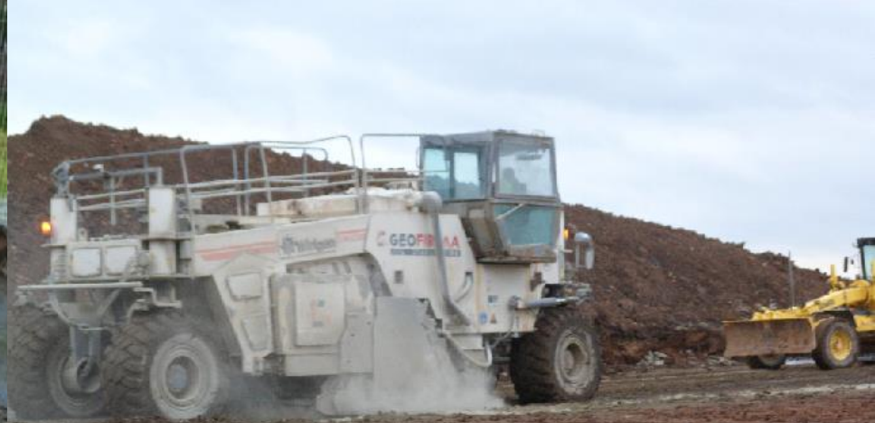
Walton on Thames Road bridge for Costain and Atkins - RoadCem turns organic mud to heavy duty cranes platforms.
