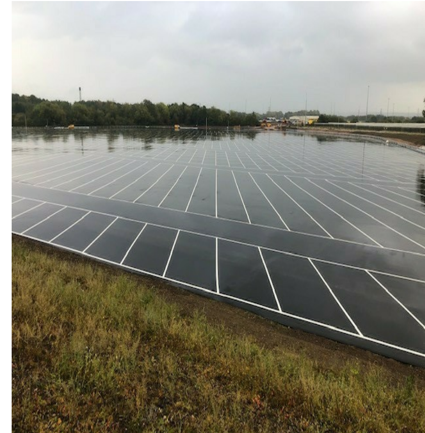
The Car Park is marked and ready for use, saving time cost and carbon. Saving 64,000 tonnes of imported stone.
