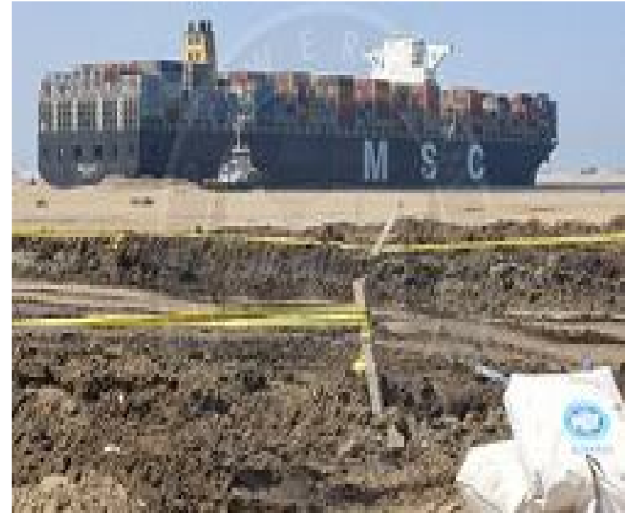
RoadCem in use for Suez Canal widening.
