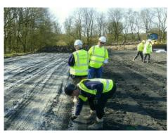
Whilst RoadCem soil concrete can be left unsurfaced, the client opted for a thin decorative layer of gravel to give additional traction during the working project.
