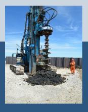
Auger drilling through the RoadCem stabilised soils was fast and safe. With no deflection and easy set up.
