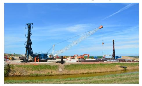
The very soft silty clays and high ground water levels presented difficult conditions to prepare an adequate working platform for the heavy plant required for the works including CFA Piling and Sheet Pile installation.
