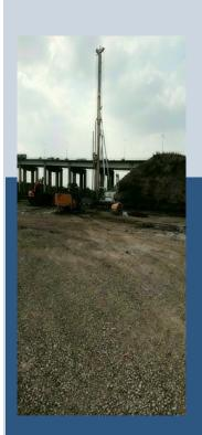
For this application a thin gravel surface was added to give extra traction and avoid any dust created during piling.
