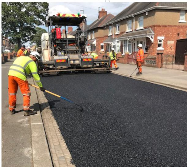
Testing confirmed the characteristic poor foundation and tar contamination. LWD's were converted to an underlying 2-4% CBR value. The challenge around the foundation issues led SPL to propose the inclusion of RoadCem.
