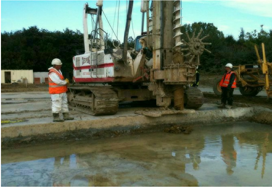
CFA Auger rig piling on the very edge of the RoadCem stabilised soil piling mat
