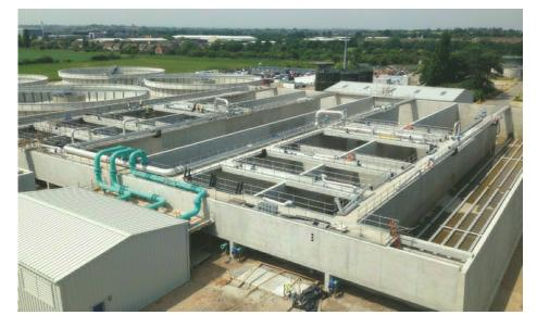
RoadCem is an innovative material successfully used by MWH to stabilize poor ground conditions and form a piling for a 75m2 concrete structure (Activated Sludge Plant) at Clay Mills WwTW.
