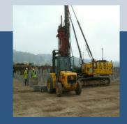
Driving piles through the RoadCem stabilised soils was fast and safe. With no deflection and easy set up.
